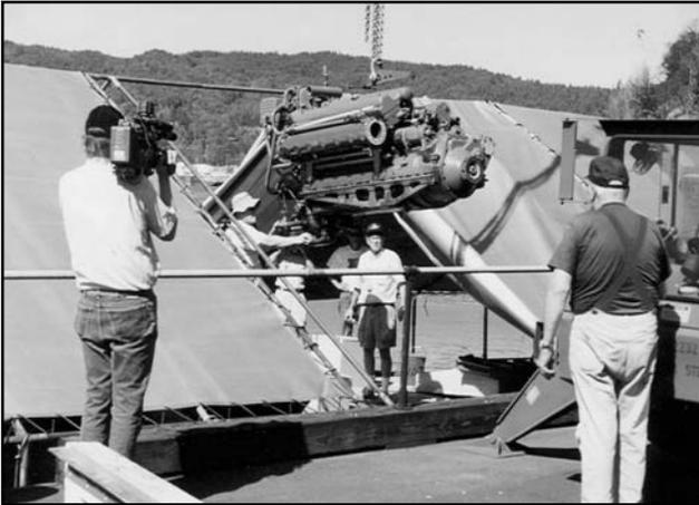
*Above: The U.S. Marine Corps provided a crane to lower PT 658's Packard engines into her engine room. All three engines were in place within three hours. Photo courtesy Save the PT Boat, Inc.*
